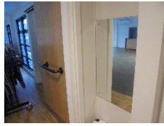
No coat hook at an accessible height
